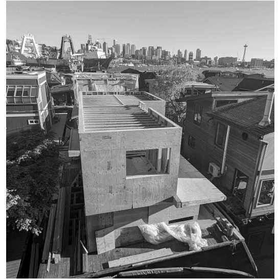
Eastlake renovation in progress by Donnally Architects and SBI Construction
